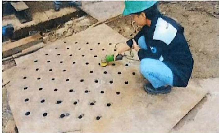
Gambar 2.1 Menggrenda Bottom Strainer Sand Filter
