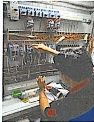
Gambar 2. 10 Continuity Jalur Kabel
