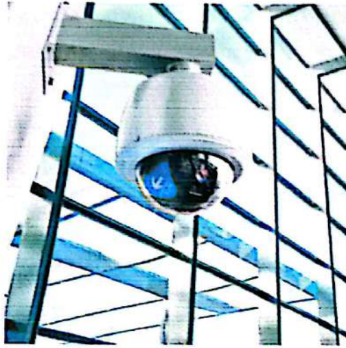
Gambar 2. 4 CCTV (Closed-Circuit Television)
