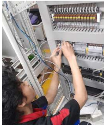
Gambar 2. 14 Menginject power Modul DI
