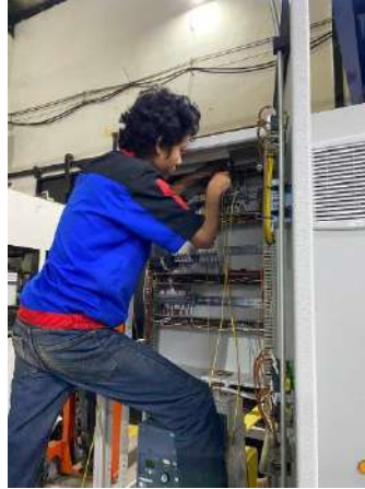
Gambar 2. 17 Proses Wiring Panel MCC & Boiller Cell 1
