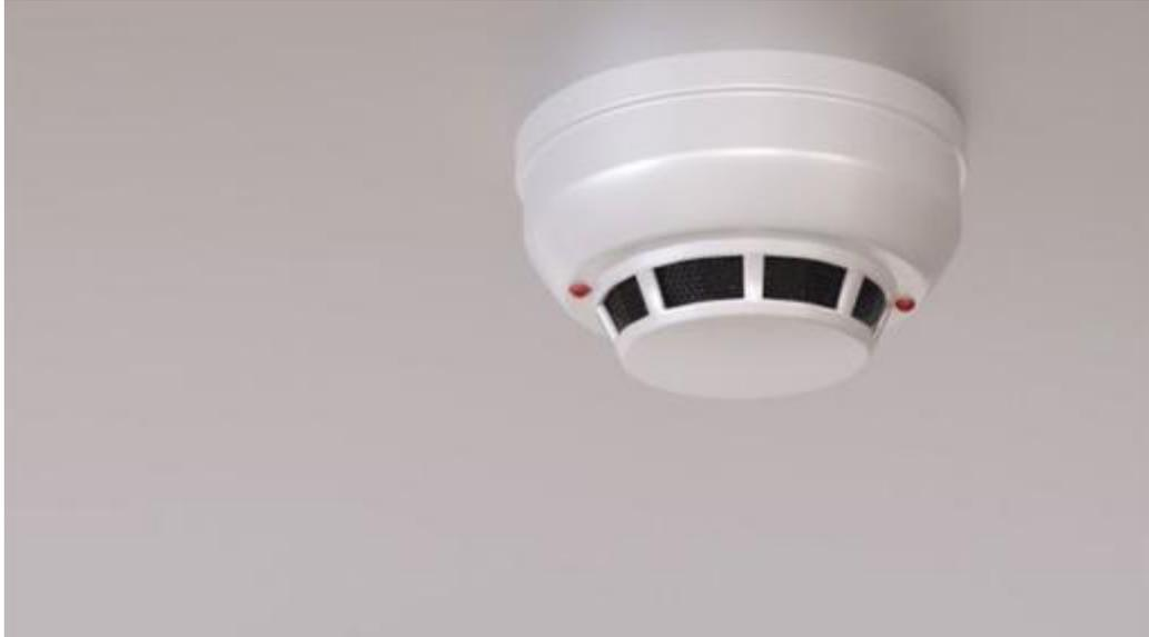
Gambar 2.7 Smoke Detector (Fire Alarm)
