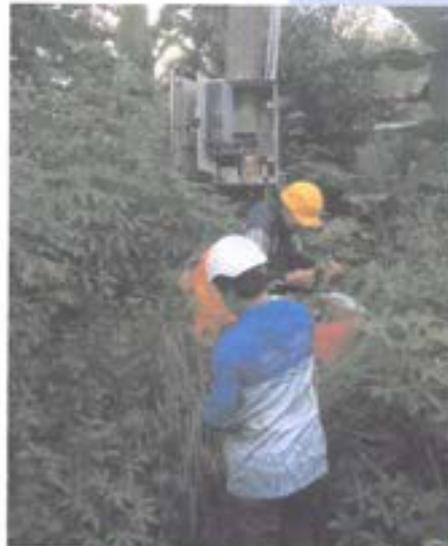
Gambar 2. 10 Pemasangan Load Break Switch (LBS) Baru
