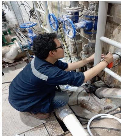
Gambar 2. 3 Tampilan Instalasi float level switch
