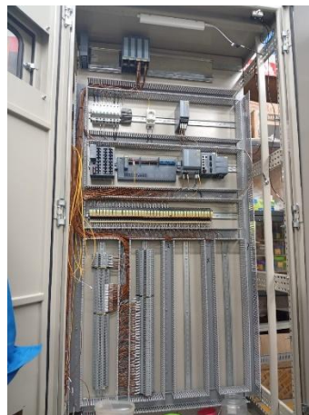
Gambar 2. 17 Proses Wiring panel PT. TAIKISHA INDONESIA
