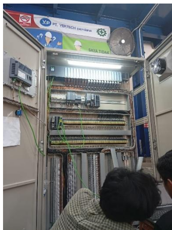
Gambar 2. 18 Proses power up dan pengecekan modul-modul PT. TAIKISHA INDONESIA
