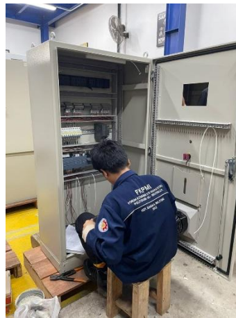
Gambar 2. 19 Proses wiring Panel PT. NUSACPTA INDONESIA
