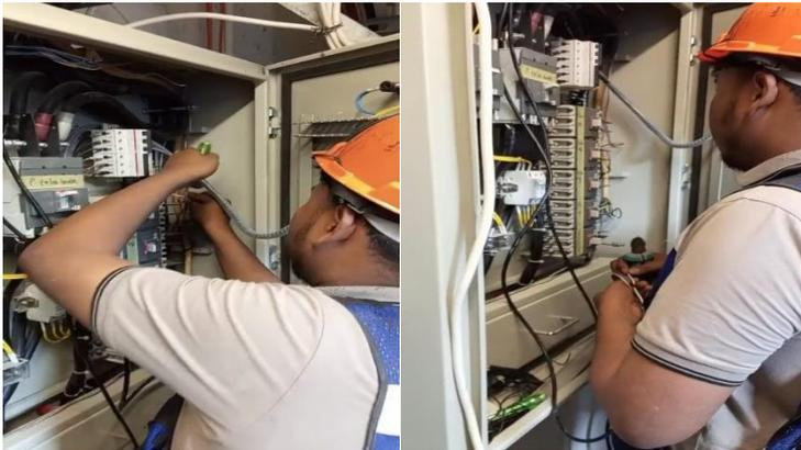
Gambar 2. 4 Terminasi Kabel Power Panel PL
