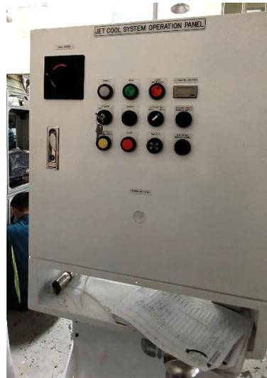
Gambar 1. 7 Jet Cool System Operation Panel
