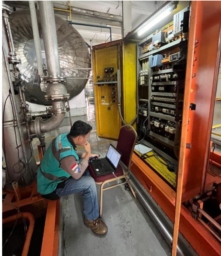
Gambar 2. 3 Proses Migrasi PLC di PT. Delta Djakarta Tbk
