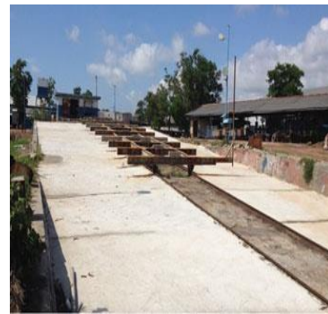
Gambar 1.10 RAIL SLIPWAY AND WINCH
