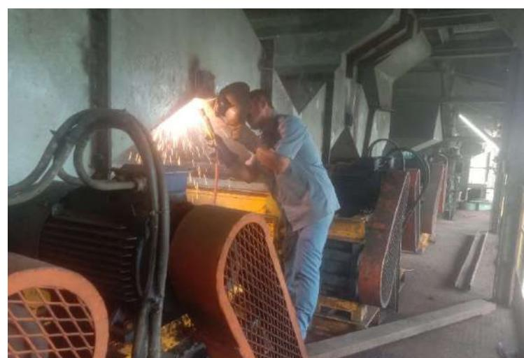
Gambar 2. 4 Pengelasan *Ducting Condisioner*
