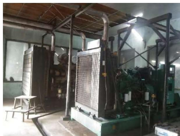
Gambar 2. 35 Mesin Gengset
