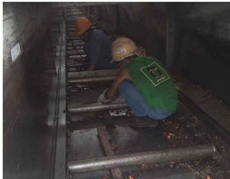
Gambar 2. 5 Pergantian *Liner/Rel Conveyor FFB*
