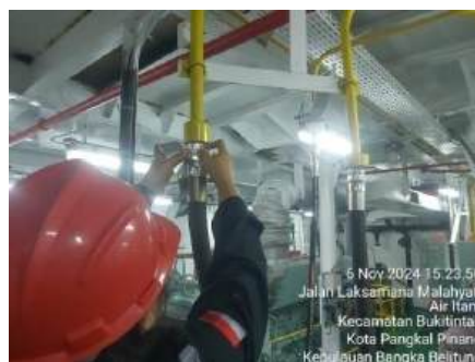
Gambar 2. 19 Pemasangan oil tap
