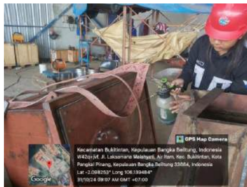
Gambar 2. 17 Air test tangki hydraulic
