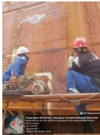
Gambar 2. 2 Vacum Test
