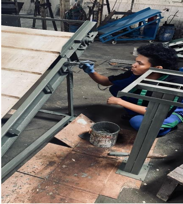
Gambar 2. 4 Proses Pengecatan Mesin Conveyor
