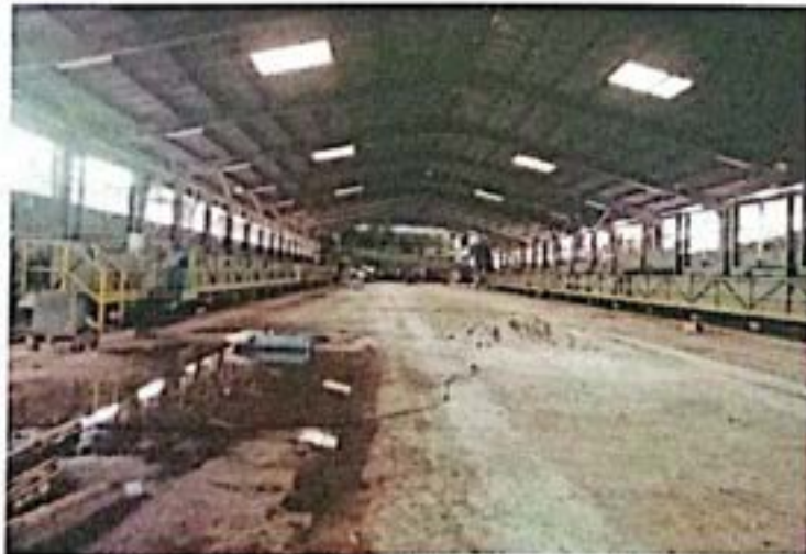
Gambar 2. 1 Pintu loading ramp
