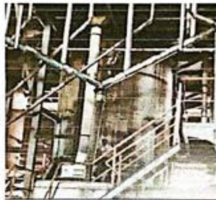
Gambar 2. 8 Sand Trap Tank
