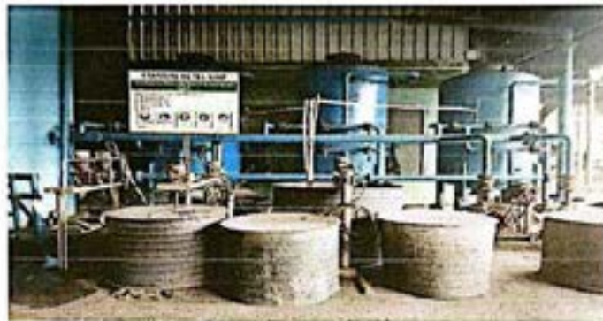
Gambar 2.23 Softener Tank
