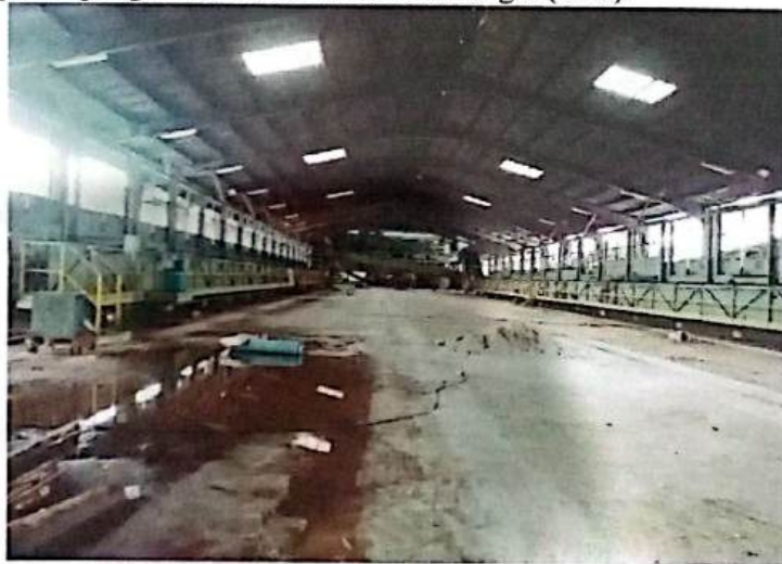
Gambar 2.1 Pintu Loading Ramp
