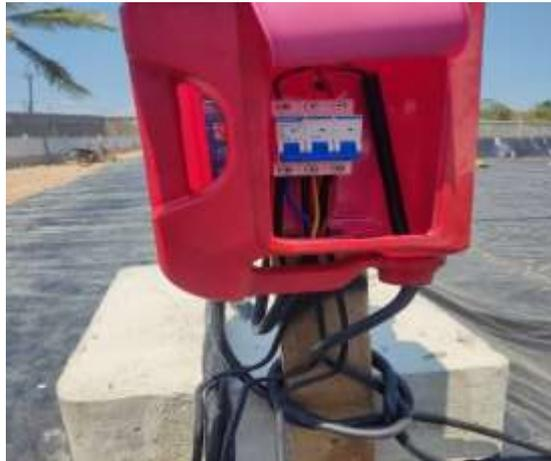
*Gambar 2. 8 Proses Instalasi MCB 3 Phase*
