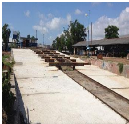
Gambar 1.1 Rail Slipway And Winch
