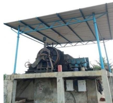
Gambar 1.2 Air Bag Slipway And Winch
