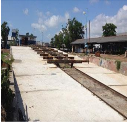
Gambar 1.2 Rail Slipway And Winch
