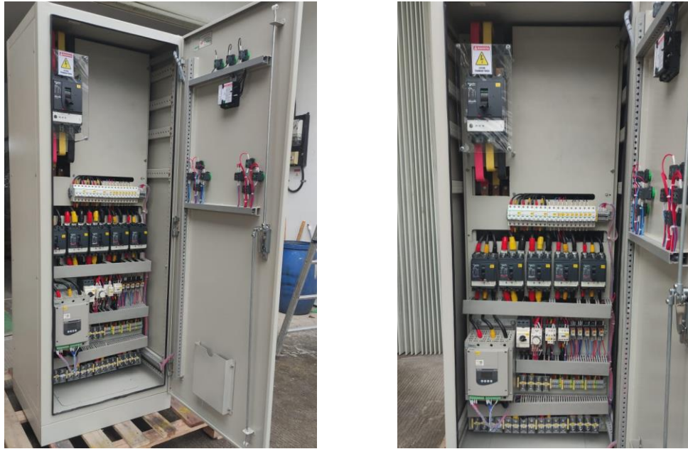
Gambar 2. 40 Hasil Akhir Panel SDP Utility 4
