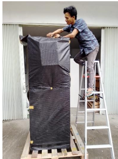
Gambar 2. 41 Pemasangan Bubble Wrap Panel SDP Utility 4
