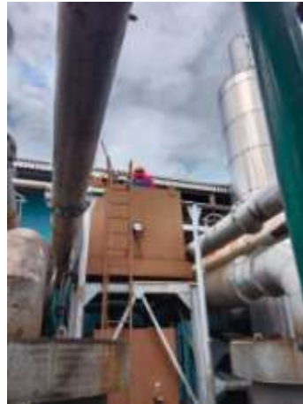
Gambar 2.10 Menguras endapan daily tank BBM
