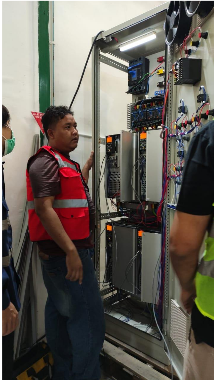
Gambar 2. 25 Panel Kontrol Cooling Water Pump PT.Rajawali Anugrah Prima
