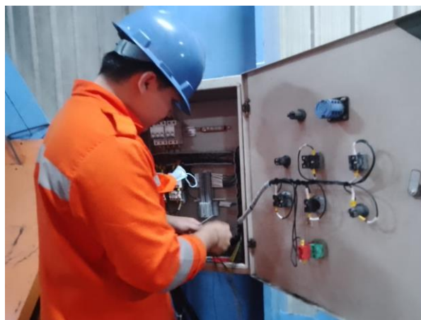
Gambar 2.4 Terminasi Panel BFC,BFD,dan BC04
