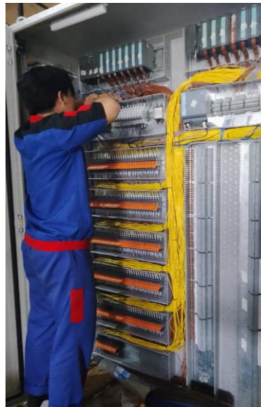
Gambar 2.2 Wiring panel
