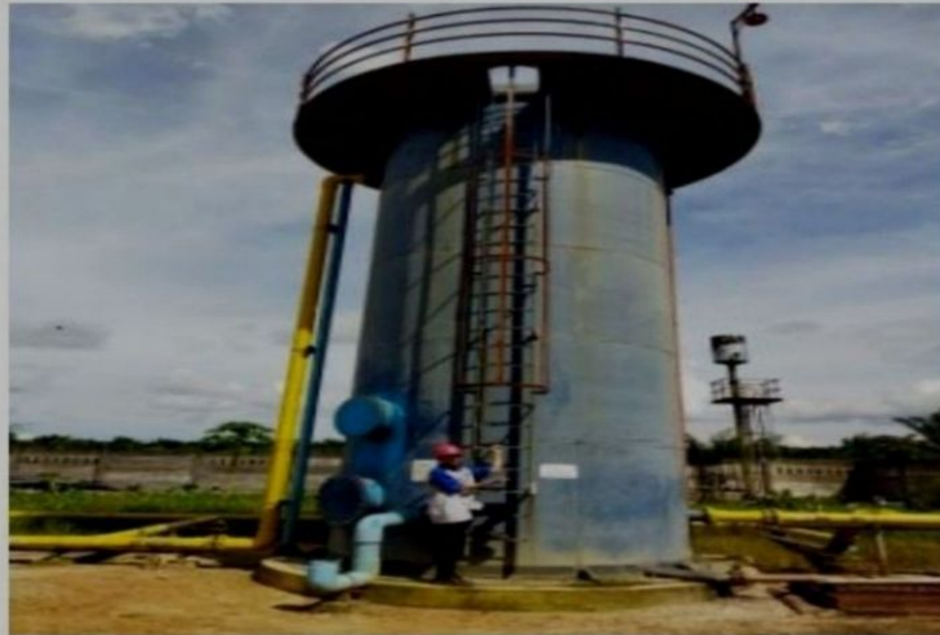
Gambar 1. 11 Wet biological filter
