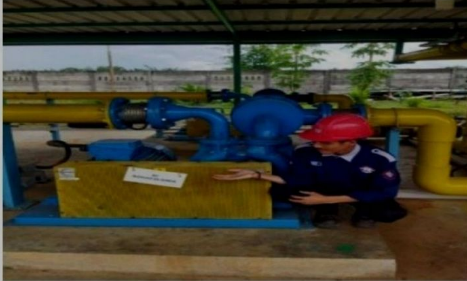
Gambar 1. 15 Biogas blower
