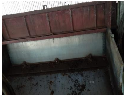
Gambar 2.2 Pintu Loading Ramp
