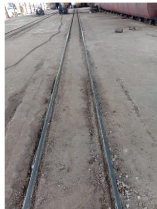
Gambar 2.8 Rel Loading Ramp
