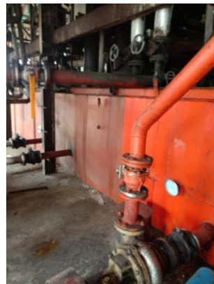
Gambar 2.25 Crude Oil Tank (COD)
