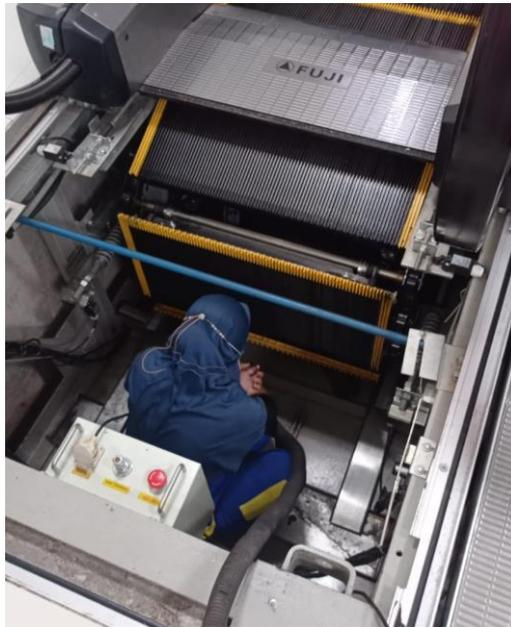
**Gambar 2.2** Pembersihan area panel kontrol eskalator
