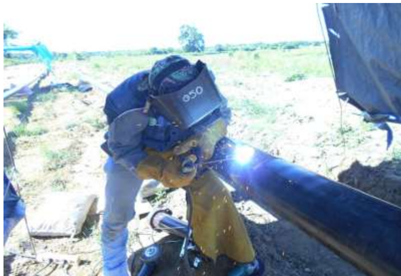
Gambar 2.7 Proses Welding Joint Pipa
