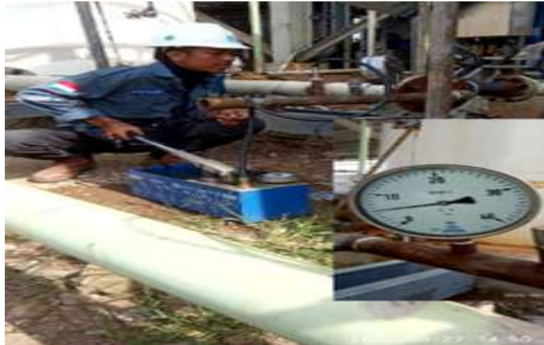
Gambar 2.12 Proses Hydrotest Pipa area SO 2 Scrubber
