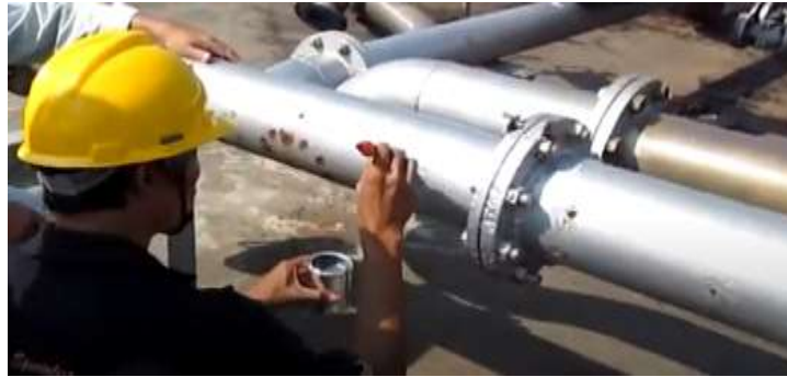
Gambar 2.5 Proses Painting Pipa
