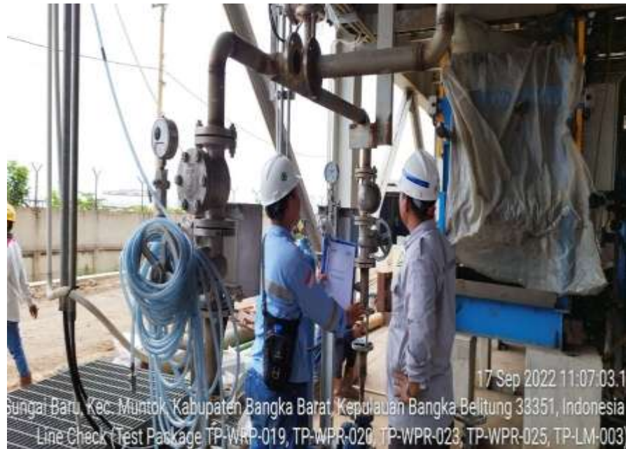
Gambar 2.16 Line Check Piping
