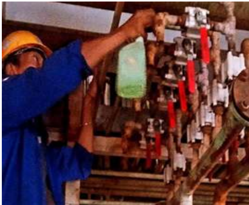
Gambar 2.11 Proses Tes Kebocoran Pipa area Furnace
