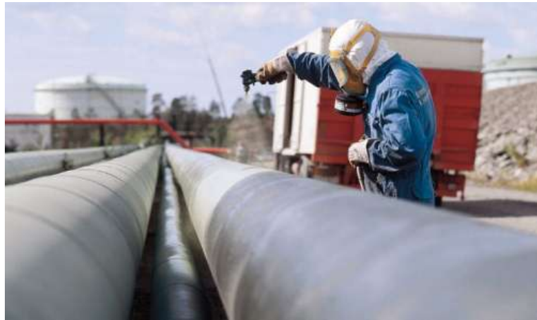
Gambar 2.4 Proses Sandblasting Pipa
