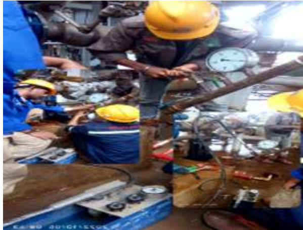
Gambar 2.13 Proses Flushing Pipa di area SO 2 Scrubber
