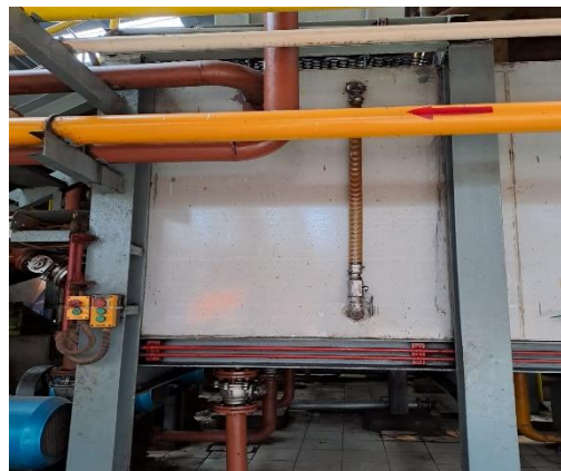
Gambar 1. 26 Dirty Oil Tank
