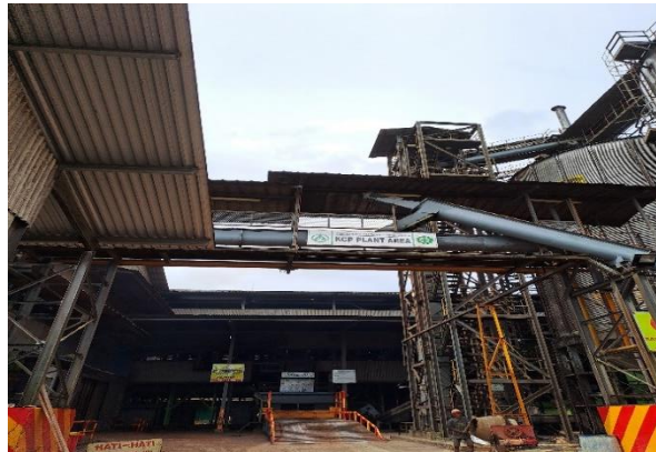
Gambar 1. 10 KCP Plant Area
