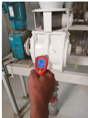
Gambar 2. 4. Mengecek suhu body airlock
