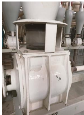
Gambar 2. 6. Mengecek kebocoran airlock
