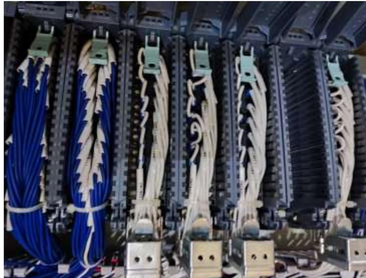
Gambar 2. 9 Wiiring Modul PLC Digital Input dan Analog Input (2 Wire Transmitter)
