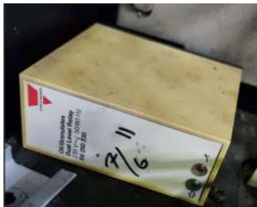
Gambar 2. 14 *Oil Level Dual Relay*
