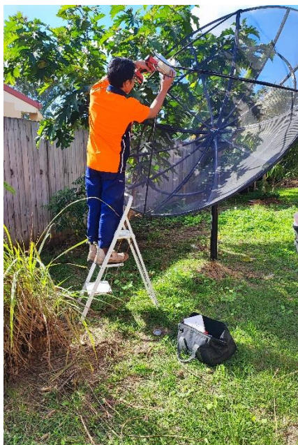
Gambar 2.6 Removing satellite television
