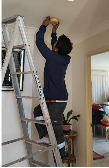
Gambar 2.10 Pengecekan fungsi alarm
