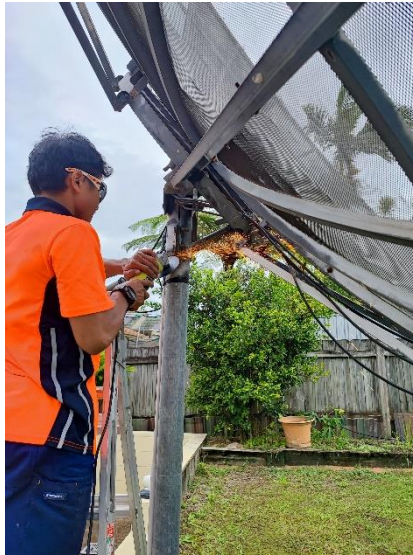
Gambar 2.5 Removing Satellite television
