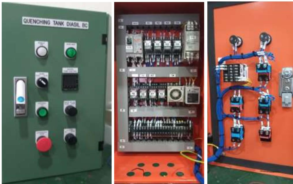
Gambar 1. 9 Box Panel *Quenching Tank Diasil BC*
