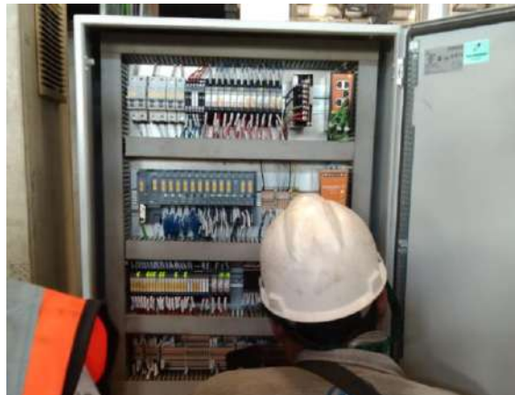
Gambar 2. 16 Re-labelling Panel Autoclave dan JB
